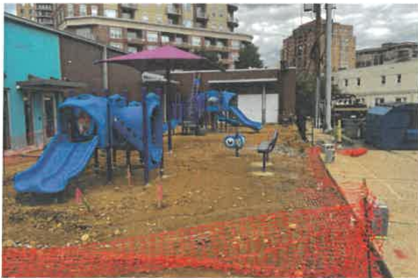
Installation of playground equipment
