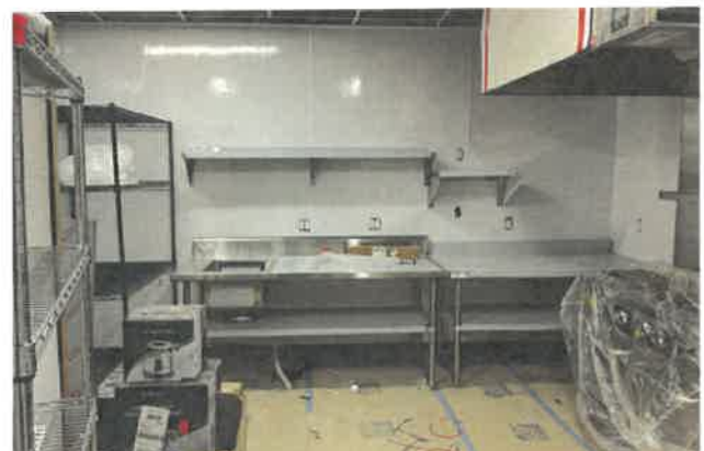
Installation of kitchen electrical
