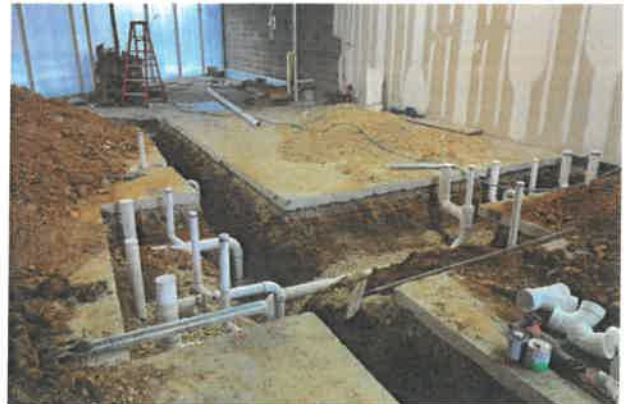
Digging trenches for plumbing
