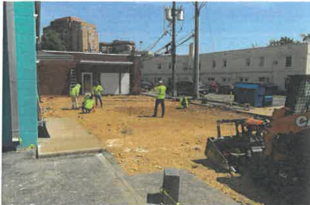
Removal of concrete
