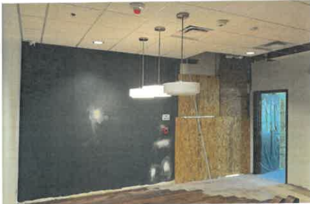
In-progress reception wall
