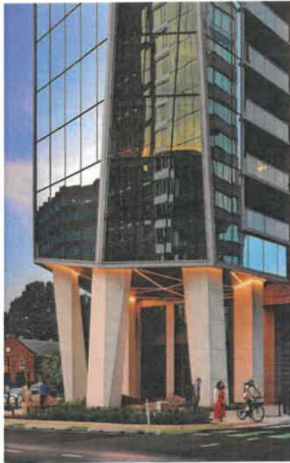
5 Chamfered Carrara Columns
