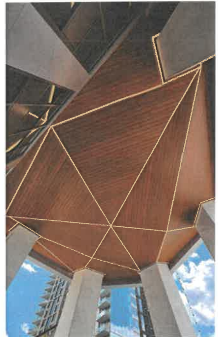
6 Chamfered Plaza Ceiling
